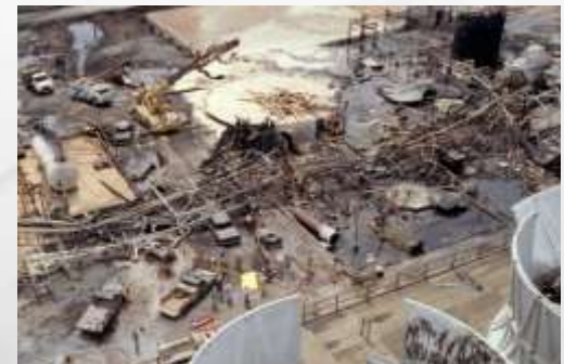
Arco Chemical (1990) 17 Dead; 5 Injured; $36 MM in damage
