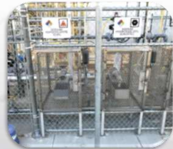
Separation of unloading connections with secure cages around connection points (Source: MGPI)
