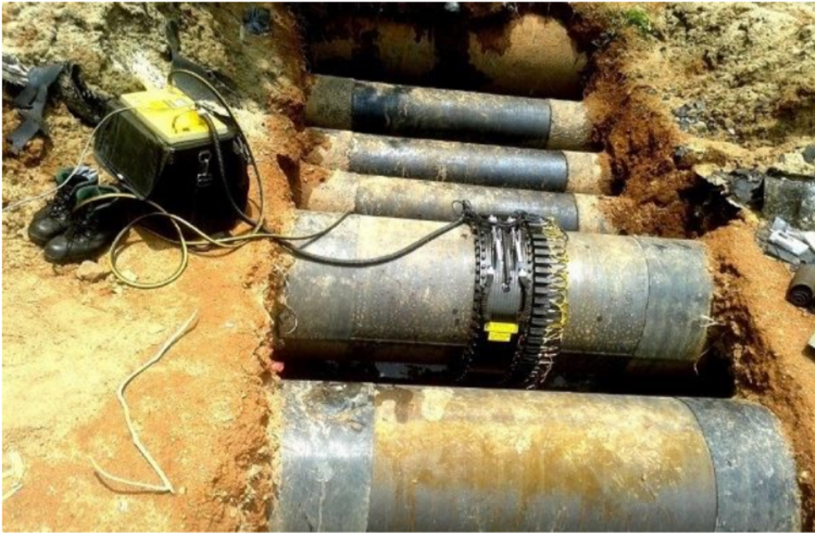
Figure 7. Applying long range ultrasonic testing to observe the situation of pipes. 11
