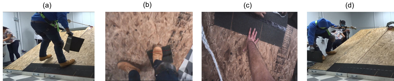
Safety incidents: (a) Near-skid; (b) Slip hazard; (c) Nail puncture hazard; d) Fall off roof
