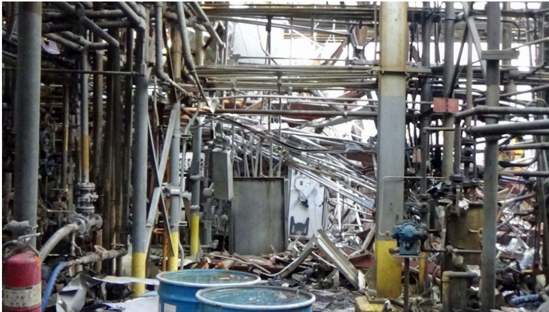
Figure 13. R2 Building (North Side). This post-incident photo shows the path KMCO workers commonly took to enter the R2 Building. With process units on the left and right, this walkway led to the entrance on the north side of the R2 Building, where emergency responders found Board Operator 2. (Credit: CSB)
