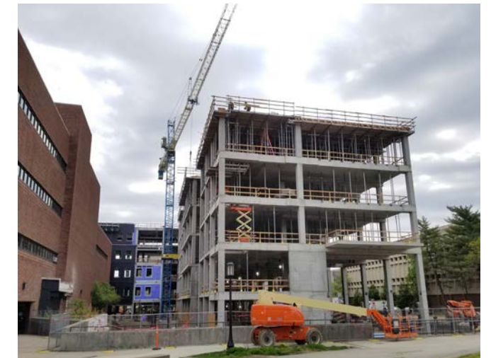
Construction progress is made in early fall 2021
