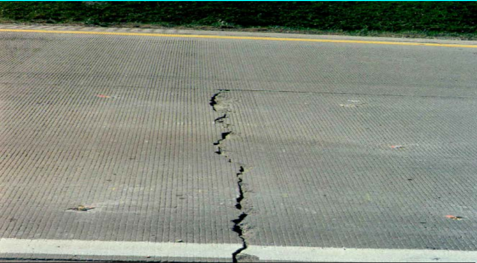
Transverse Cracking
