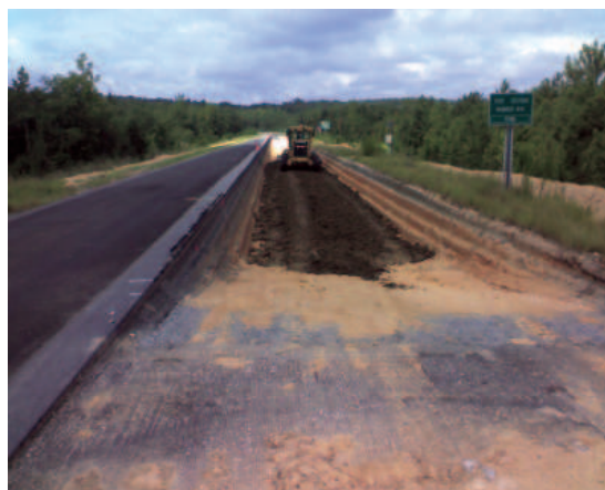
Figure 2. Installing Soft Subgrade
