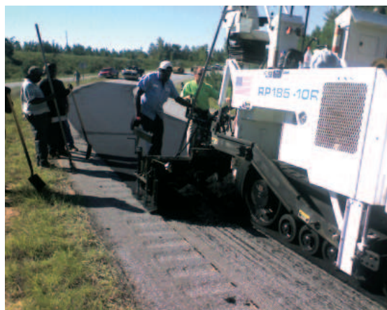
Figure 3. Paving E5 with 45% RAP
