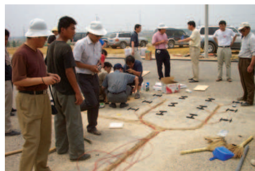
Figure 4. Asphalt Strain Gauges During Construction in May 2005.
