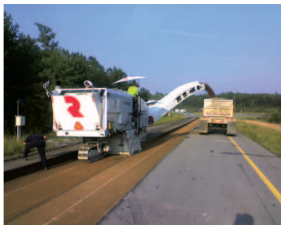
Figure 1. Milling N1 and N2
