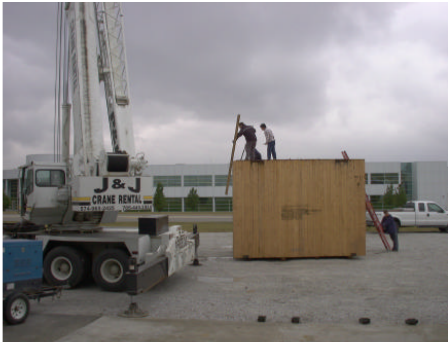
October 28, 2004 – first test rig and three wheel loaders arrived from Germany
