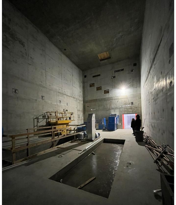
*ZL9's test cells are an astonishing 34 feet tall. The three rectangular inlets will deliver high-pressure heated air.*
