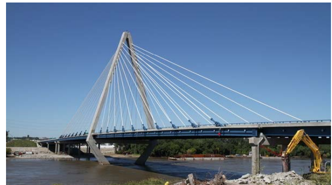
▶ Christopher S. Bond Bridge
