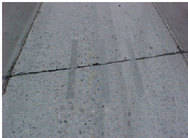
Dowel bar retrofit across a crack (Wilson and Toepel, 2002)
