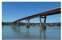
• McMillan Creek Bridge, City of Prince George, BC: Design Engineer for the detailed design of the bridge structure. The bridge consists of a pile-supported 21.2 m span. The superstructure is comprised of single cell prestressed boxes supporting a 200 mm thick cast-in-place High Performance Concrete (HPC) deck. Access from the planned fishing park trail north of PG Pulpmill Road to the Nechaco River is provided with a 2.5 m wide reinforced concrete path under the bridge.
