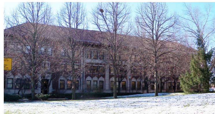
View of ABE Building Looking South
