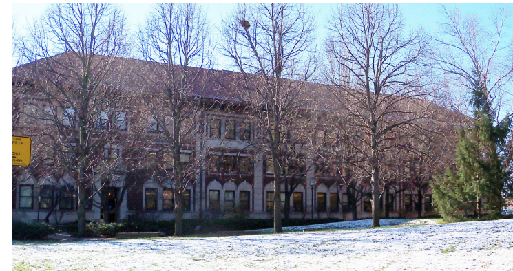
View of ABE Building Looking South
