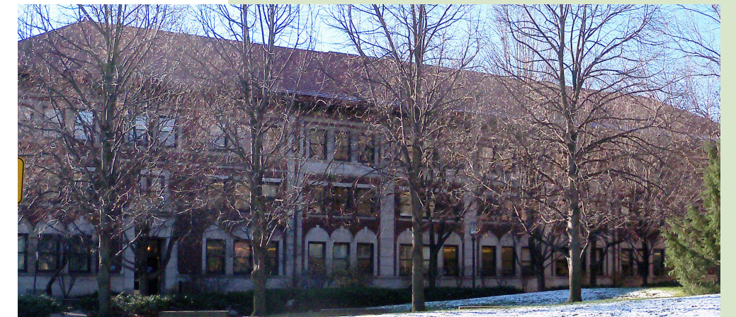
Existing ABE Building Looking South
