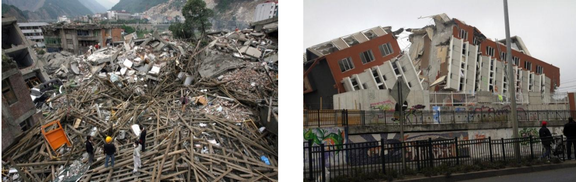
Figure 1.1: Earthquake damage in (a) Sichuan Province, China and (b) Santiago, Chile
