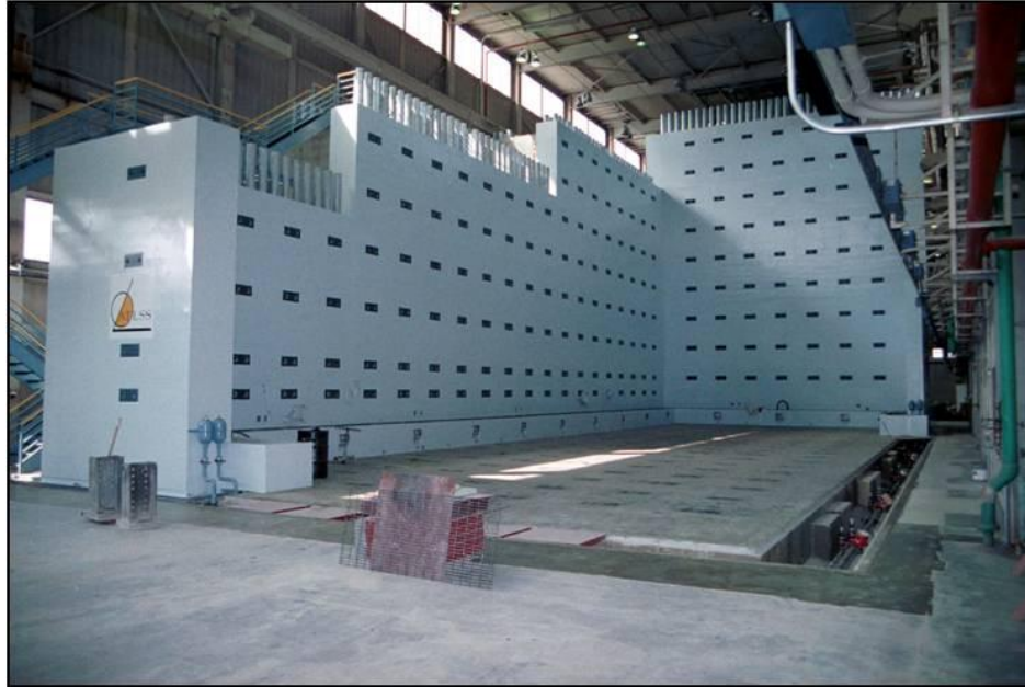
Figure 4.7: NEES@Lehigh Testing Facility and Reaction Wall
