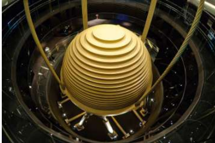
Figure 1.5: TMD installed in Taipei 101 in Taiwan
