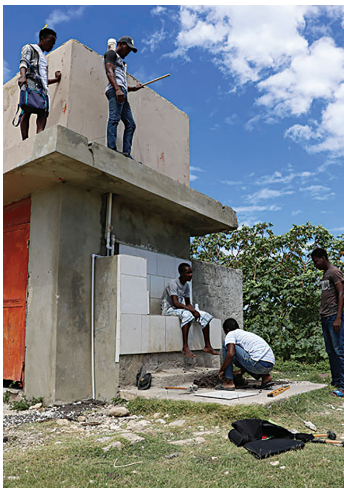
Plumbing class students McKinley and Jude (top) install plumbing for drinking water while tiling class students Louis Mark, Kerson and Orlando (bottom) practice laying tile.
