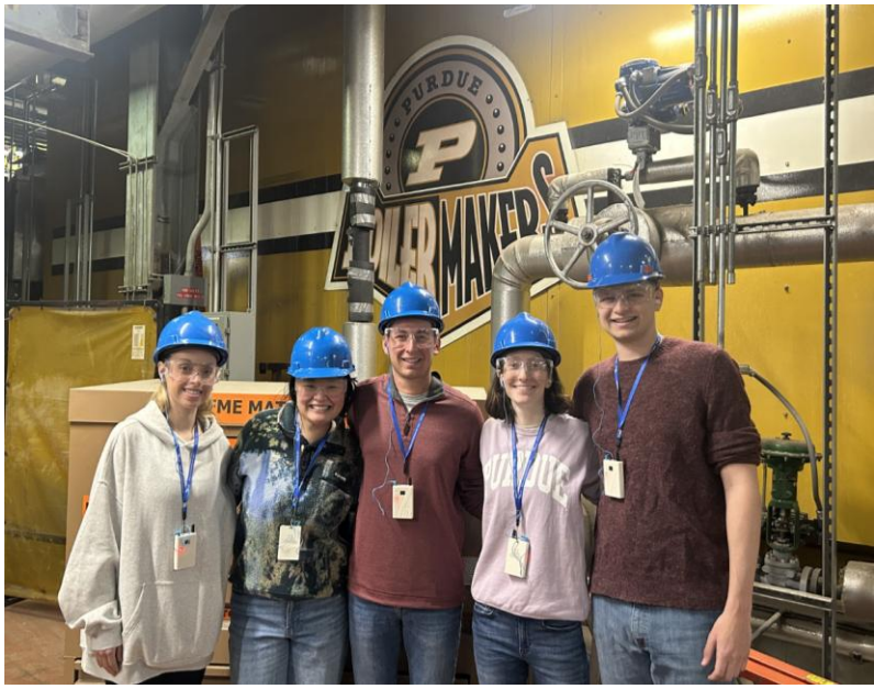
Purdue University Wade Utility Plant
