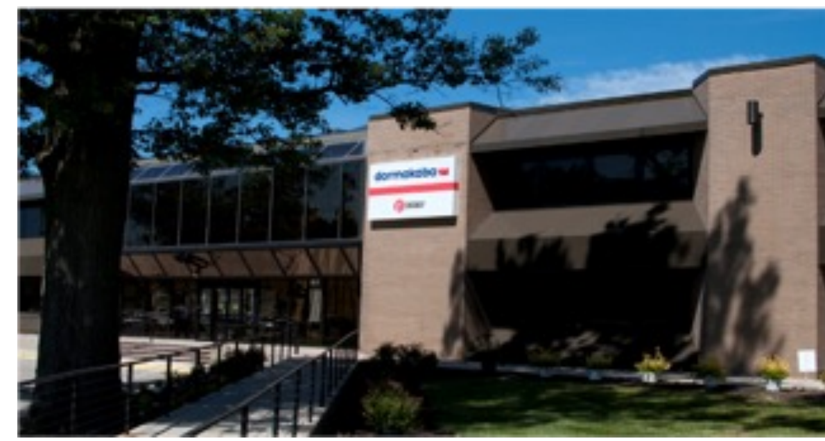
Facility located in Indianapolis, IN
