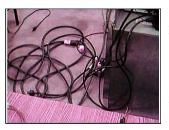
installations and must be addressed through upgrades to the building wiring systems. Extension cords should be no less than 16 gauge wire. Only "SO" type rubber covered type cord is approved. NO "ZIP cord" or "Home" type cords are allowed. Students must not attempt electrical repairs. Report problems to the shop!
