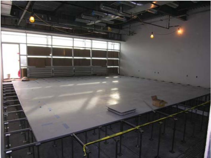
One of four rooms that comprise the Living Labs on the third floor that will house the graduate student work areas.
