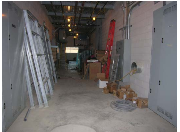
The basement hallway.
