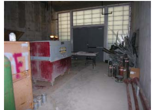
One of the four engine test cells.
