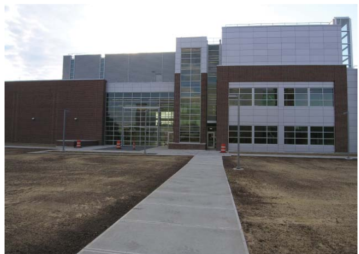
View from west side of building
