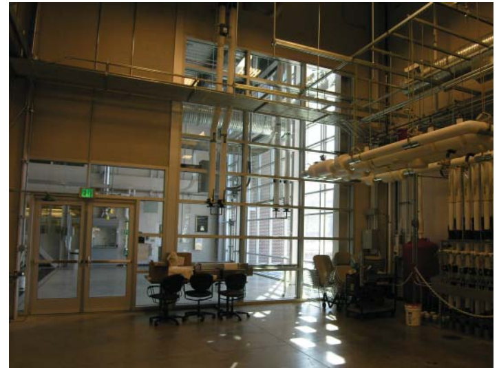
West Thermal Sciences Wing looking at High-Bay Laboratory
