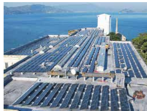
Alcatraz Island is now outfitted with a solar-powered microgrid. The 305-kW photovoltaic array installed atop the cellhouse building displaces diesel-fueled electricity. (Photo courtesy of National Park Service.)
