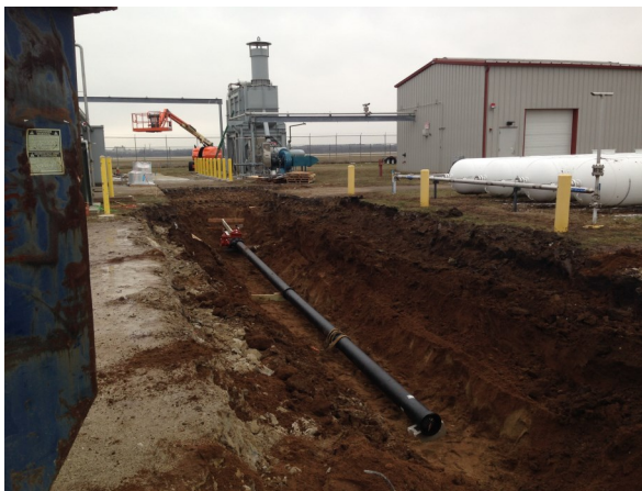
Water line installed for modified HPL. Amazingly, test operations are still going on. (1-30-16)
