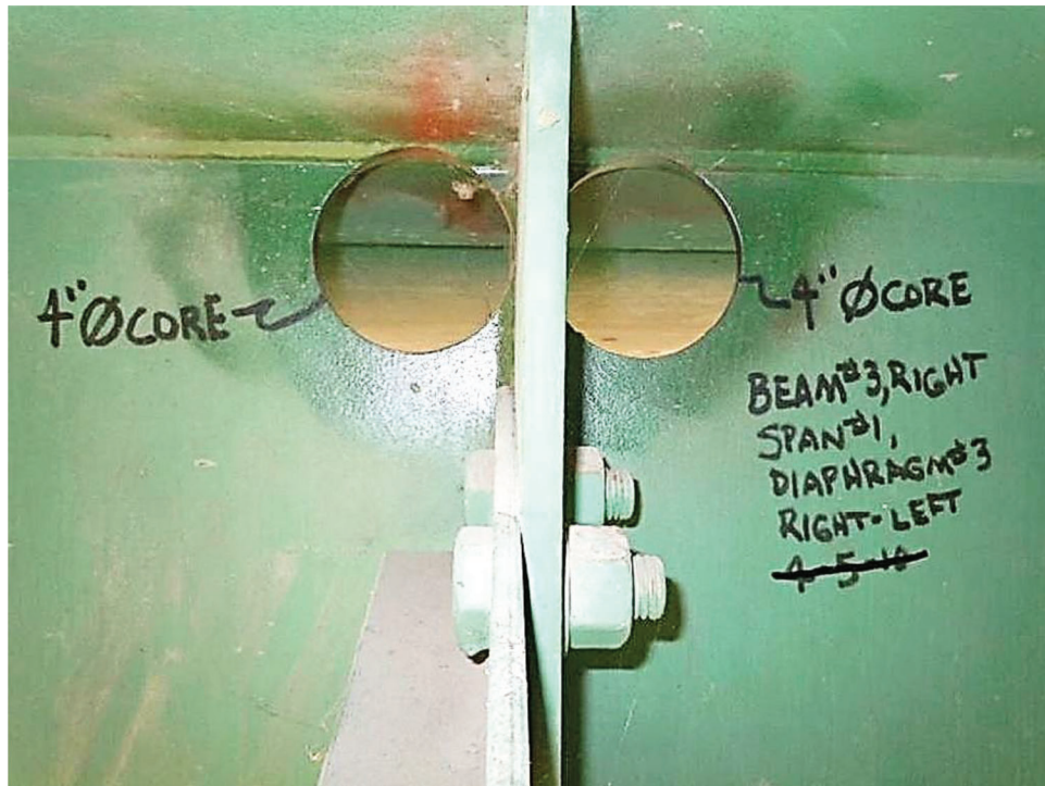
Figure 6.11 Large-hole retrofit – note interception of horizontal and vertical weld toes (Photograph courtesy of Iowa DOT).
