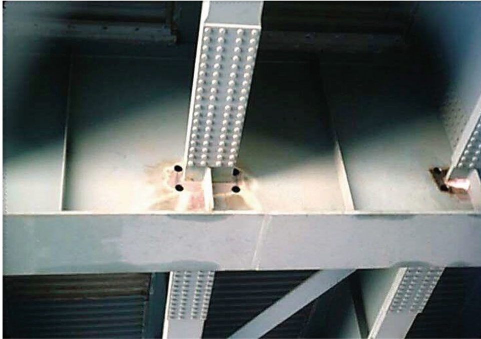
Figure 6.38 Completed dog-bone retrofit on a web penetration detail.
