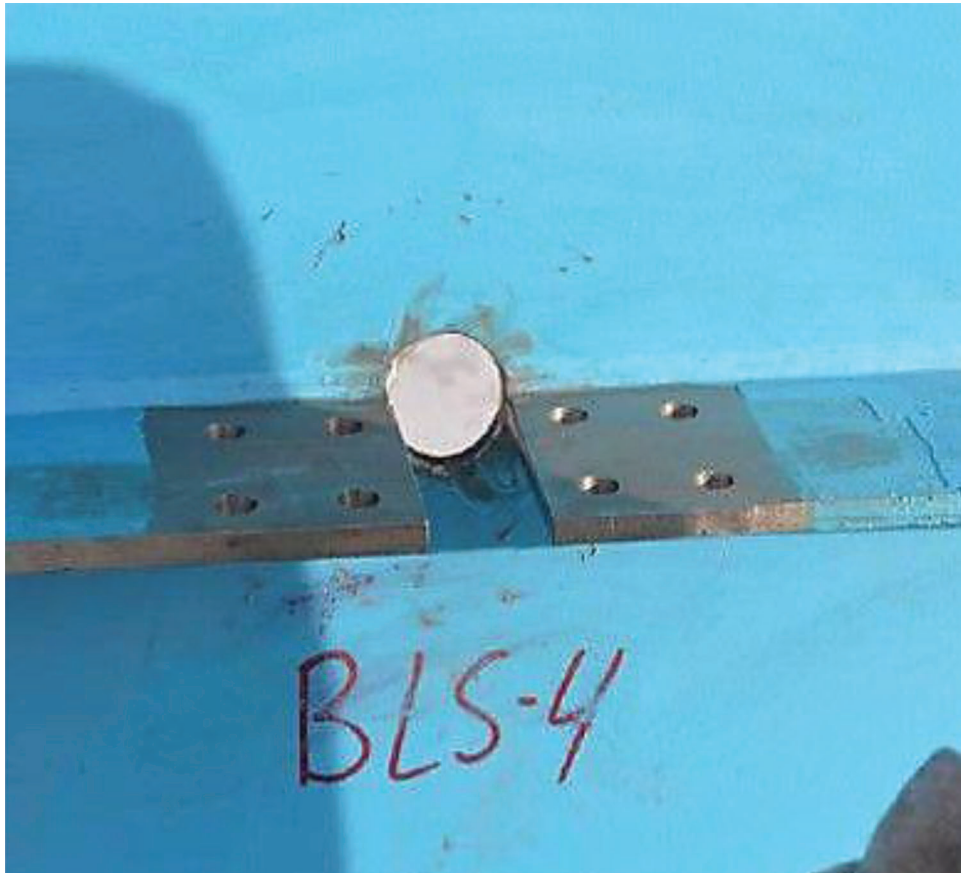
Figure 7.29 Finished retrofit with drilled holes for optional bolted splice.
