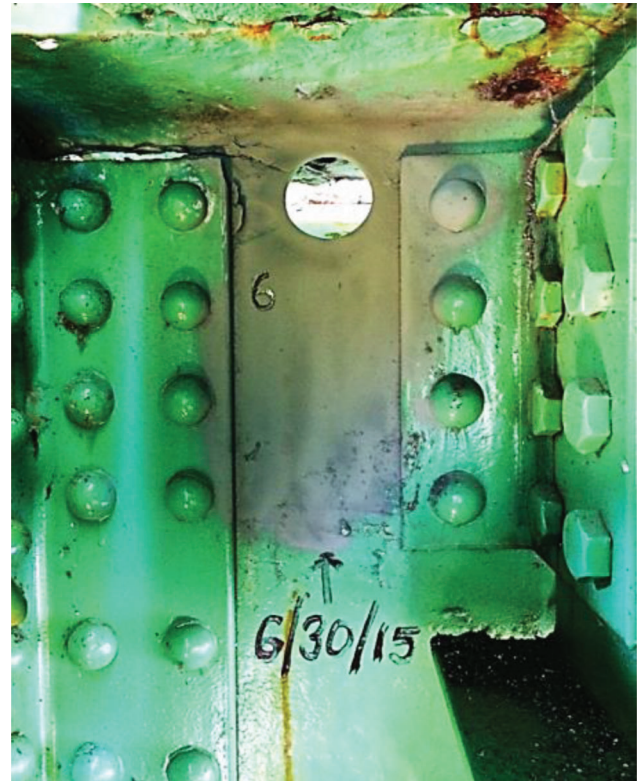
Figure 6.20 Finished repair with zinc-rich paint.
