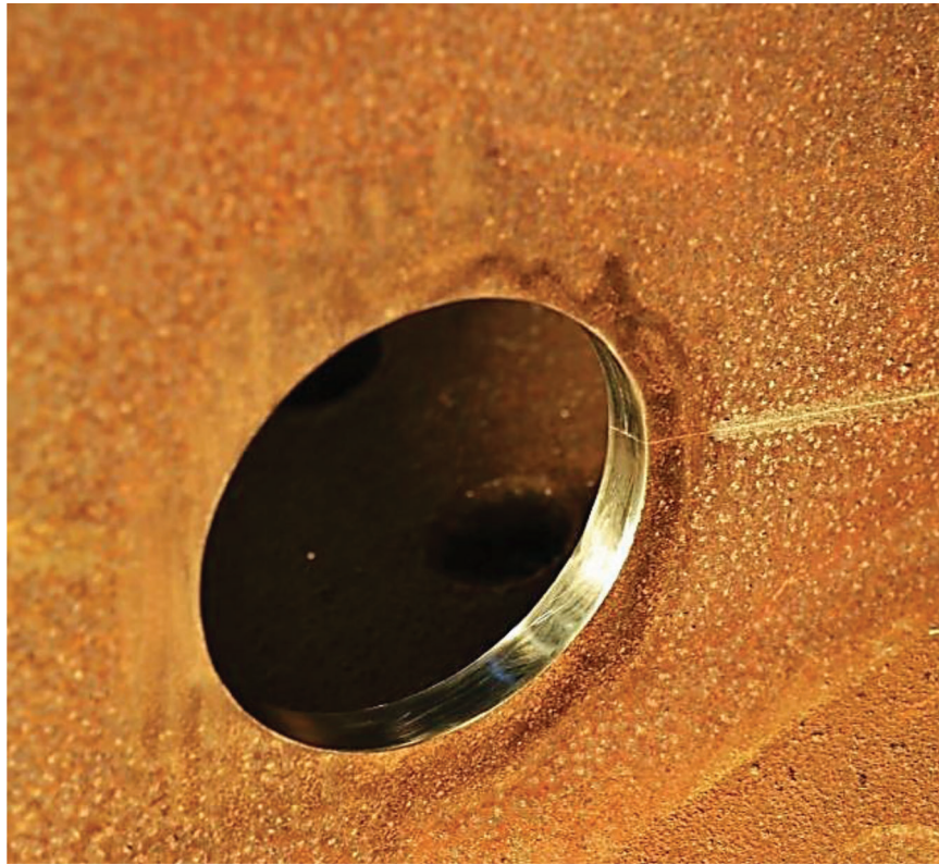
Figure 4.9 Example of finished crack arrest hole prior to painting.
