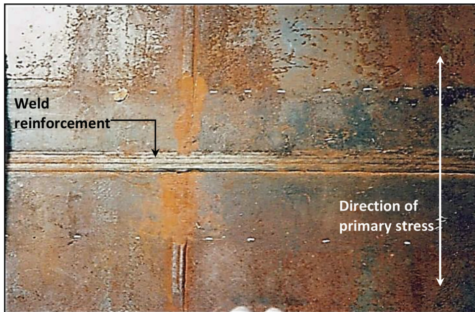
Figure 5.31 Category C transverse groove weld.
