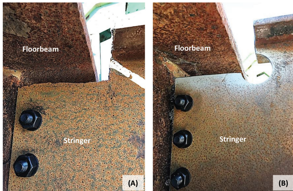
Figure 5.13 Before (A) and after (B) pictures of cope transition retrofit.
