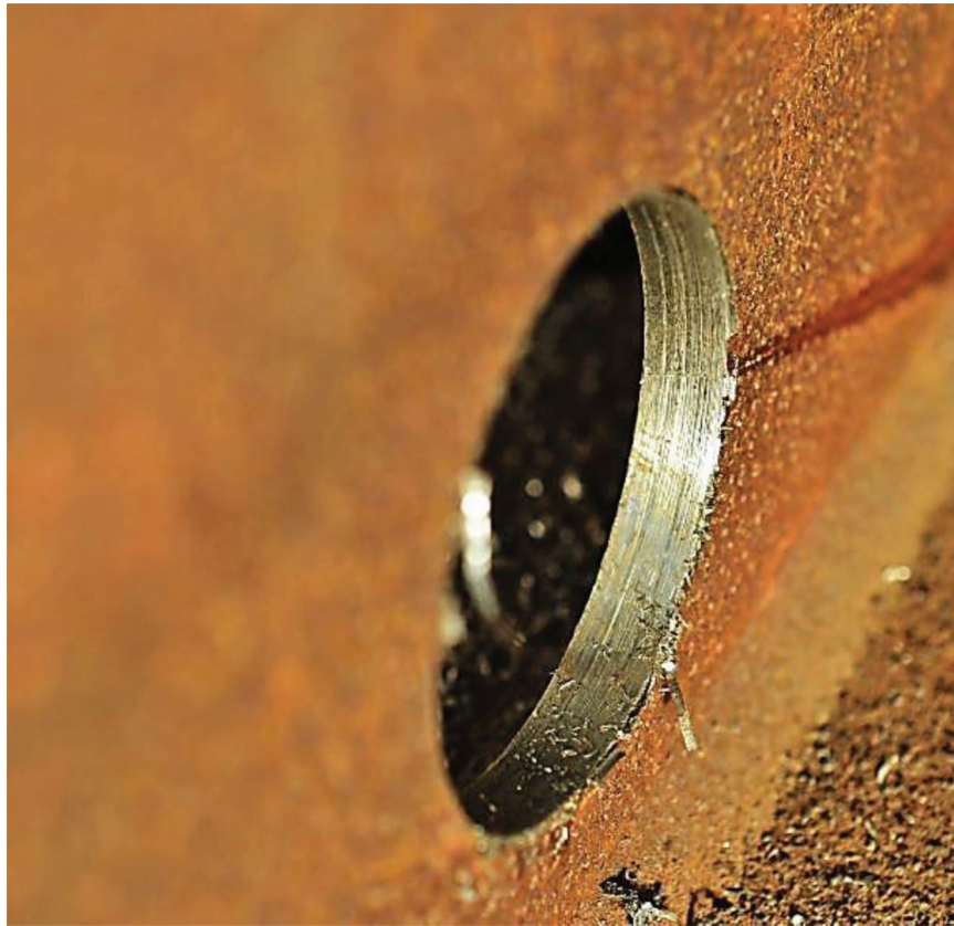
Figure 4.6 Drilled hole showing rough edges and burrs.
