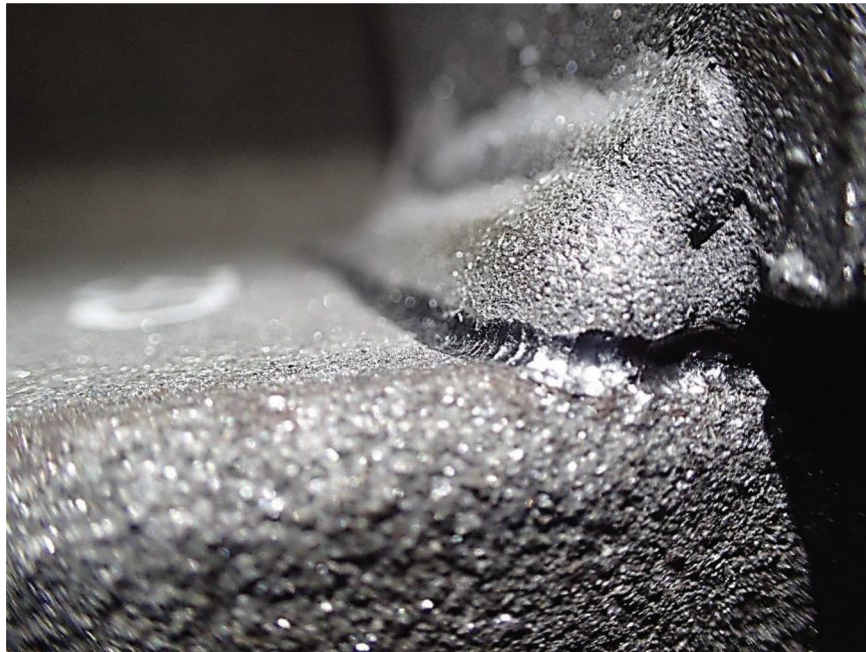
Figure 4.17 Appearance of properly treated weld toe using UNP method.
