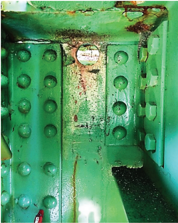
Figure 6.19 Drilled hole prior to sanding edges.
