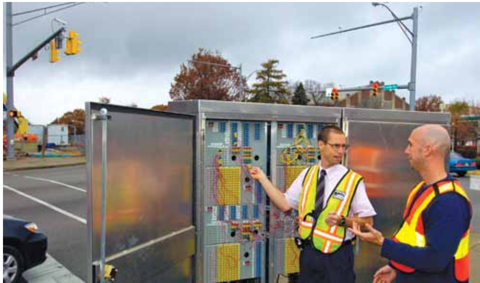
Darcy Bullock, from left, professor of civil engineering, and Edward J. Smaglik, a former postdoctoral research associate, discuss information provided by detection equipment at an "instrumented intersection." The engineers are using the system to test specialized detection and control software algorithms designed to help improve the safety and efficiency of traffic flow. (Purdue News Service photo/David Umberger)
