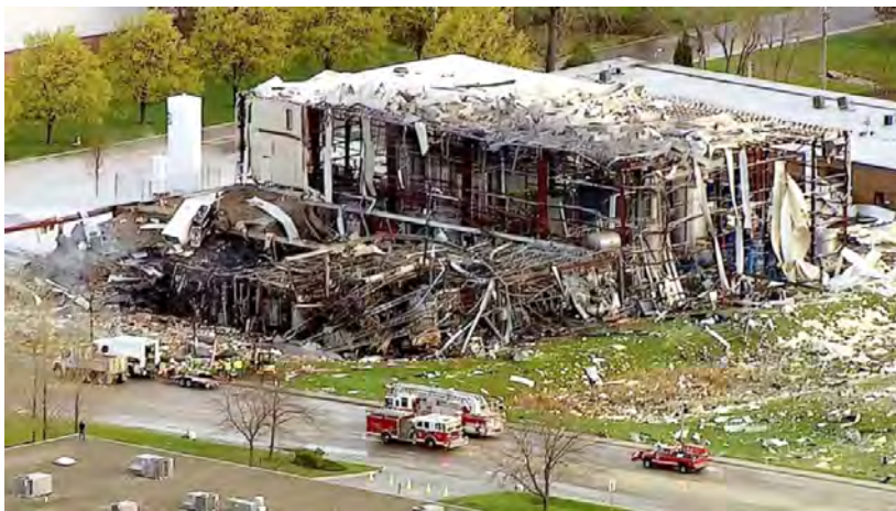
An explosion at AB Specialty Silicones facility in Waukegan, Illinois on May 3, 2019 killed four workers and caused extensive damage. The incident appeared to have been caused by the unanticipated production of flammable hydrogen gas, which combusted.
