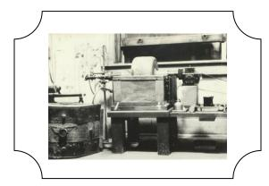
Above: One of the earliest pieces of equipment used in R.N. Shreve's work in 1932. A wrought iron ball mill used for the preparation of sodium amide by Abraham H. Goodman (M.S. '33). **Right:** The first distillation column for R.N. Shreve's research
