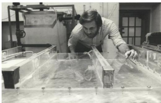
From 1970 to 1978 R. Neal House performed important research on the flow characteristics of two-phase systems using a specially constructed channel; the research was supported by NSF (1978 picture).
