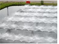
A shallow, extensive canal system provides the condenser discharge water increased contact with the atmospheric air allowing it to cool before reentry to the condenser.
