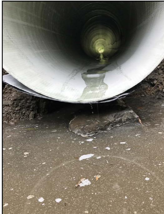
Cutting materials created during new CIPP cutting
