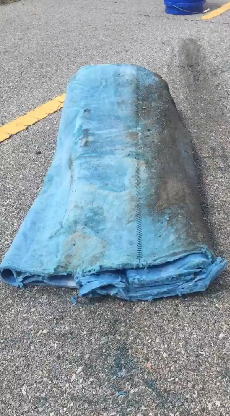
Uncured PET felt resin tube before steam curing
