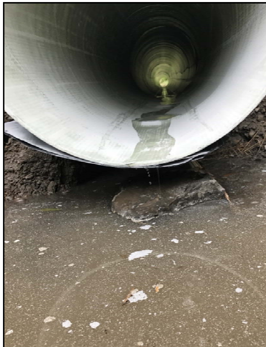
Cutting materials created during new CIPP cutting
