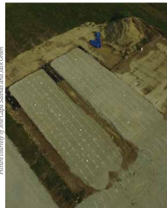
**In summer 2020**, a team of graduate and undergraduate students assisted in the construction of two testing strips at the Purdue Center for Aging Infrastructure (CAI) Steel Bridge Research, Inspection, Training and Engineering (S-BRITE) Center. The project, aimed at developing guidelines for control of the properties of aggregate drainage layers used in pavement structures, is funded by the Indiana Department of Transportation (INDOT).
