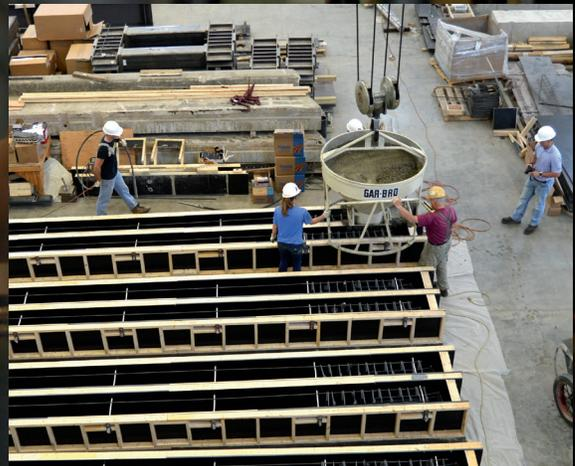
Above, Rebecca Glucksman, CE graduate student, and Harry Tidrick, Bowen Lab manager, place concrete into the formwork. Professor Robert Frosch leads the research team that is testing and codifying splice-length requirements when using high-strength steel for seismic and non-seismic applications.
