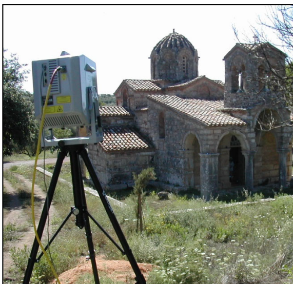
Static Terrestrial Laser Scanning
