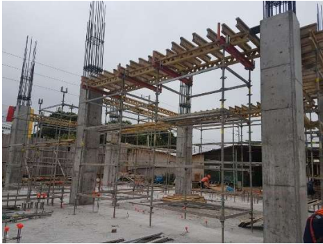
Figure 3.7. Column poured until beam bottom
