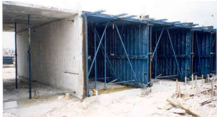
Figure 3.20. Monolithic structure with tunnel formwork
