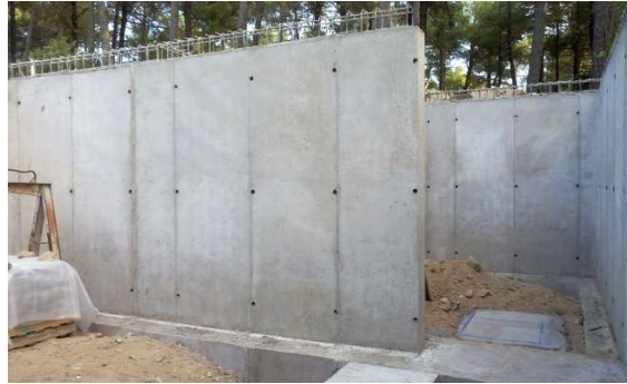
Figure 3.8. Wall poured until slab bottom
