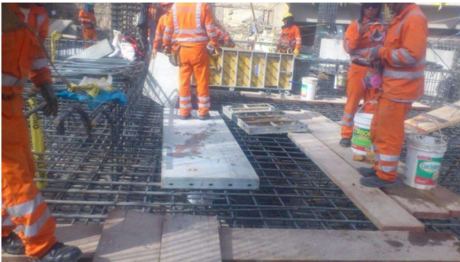
Figure 2.9. Formwork element used as a work platform
