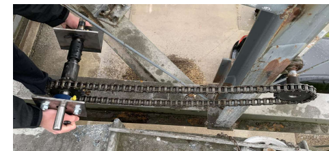
Testing of Motor Mount on Overhead Grain Bin
