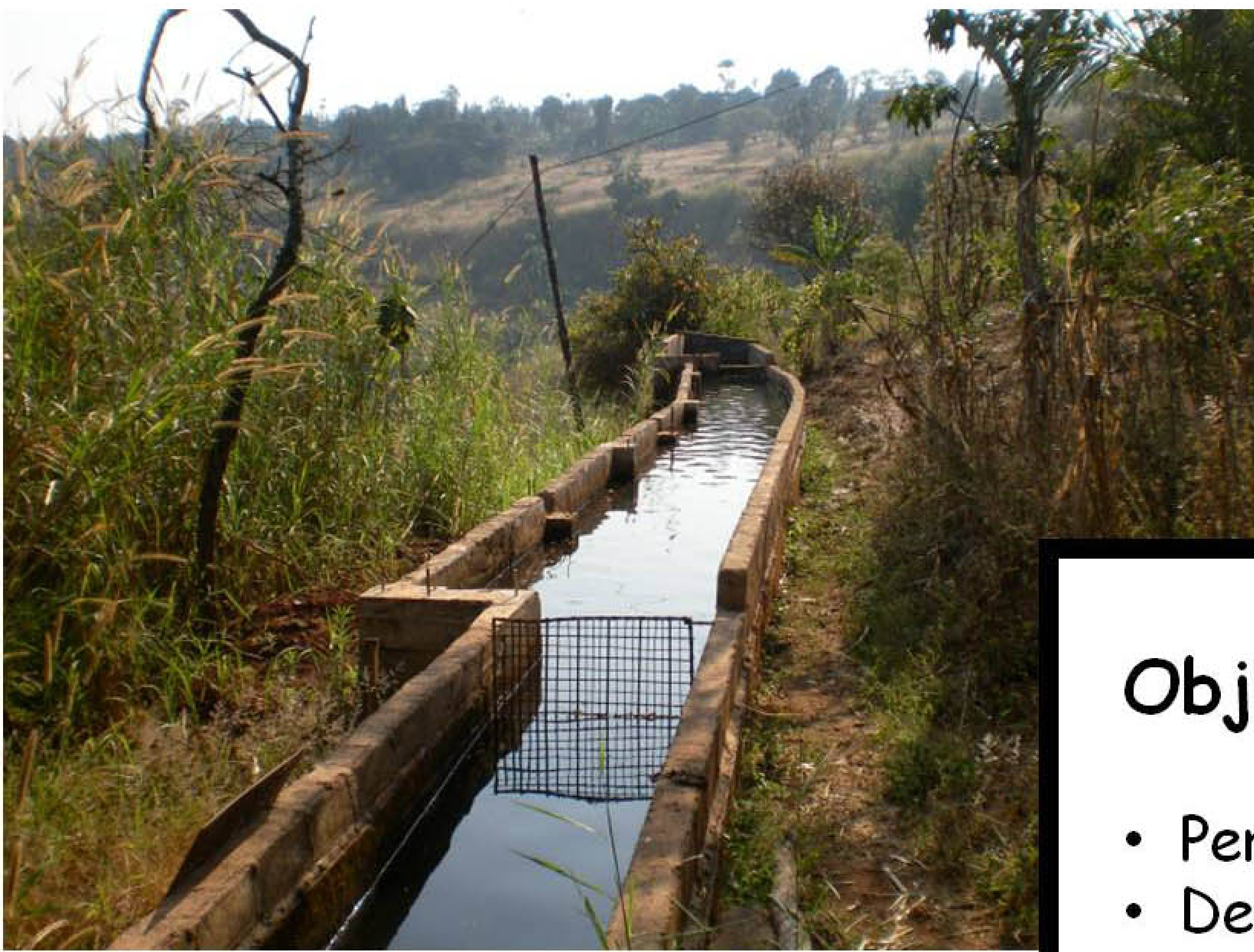
Figure 1. The canal leading water from the source to the penstock.
