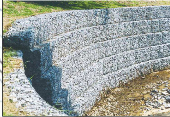
Alabama NRCS example of gabion structure ( www.al.nrcs.usda.gov )
