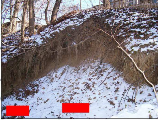
January 2007 photograph highlighting locations of seeping water
