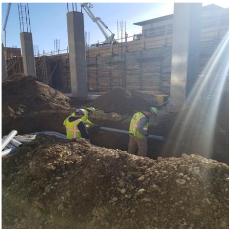
Electrical Site Work
