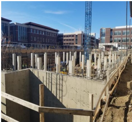
Concrete from NE corner facing SW
