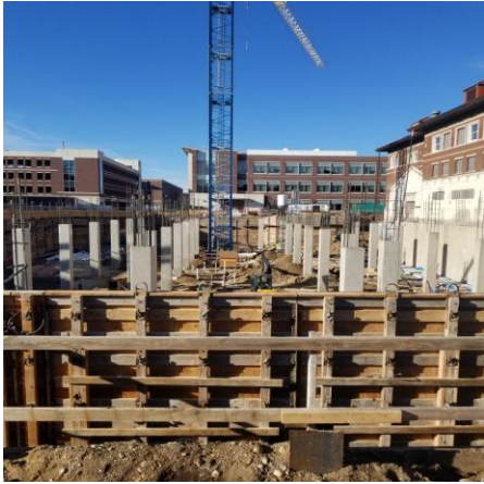
Concrete Work – facing West
