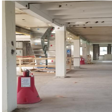
Renovation Building – 2 nd Floor facing West
