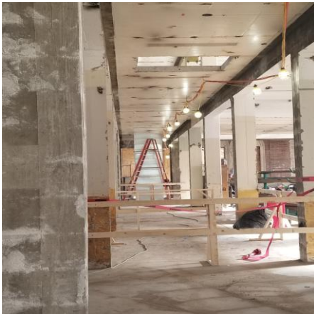
Renovation Building – 1 st Floor facing East
