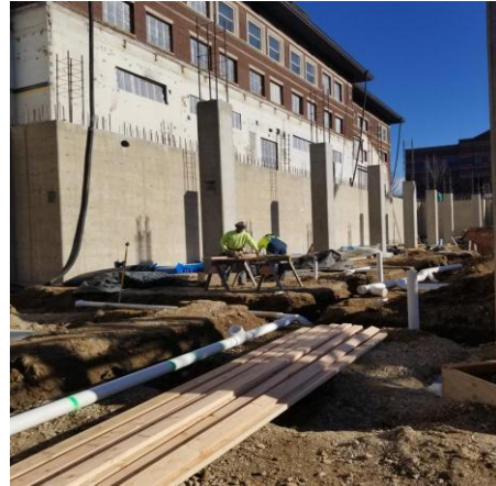
Concrete Wall and Columns – North Wall
