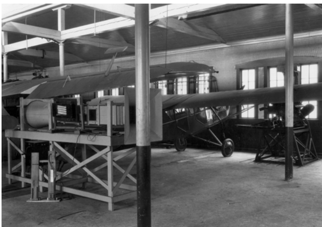
Figure 3 Aeronautics laboratory with wind tunnel, Curtiss Robin aircraft, and engine, May 1930.
