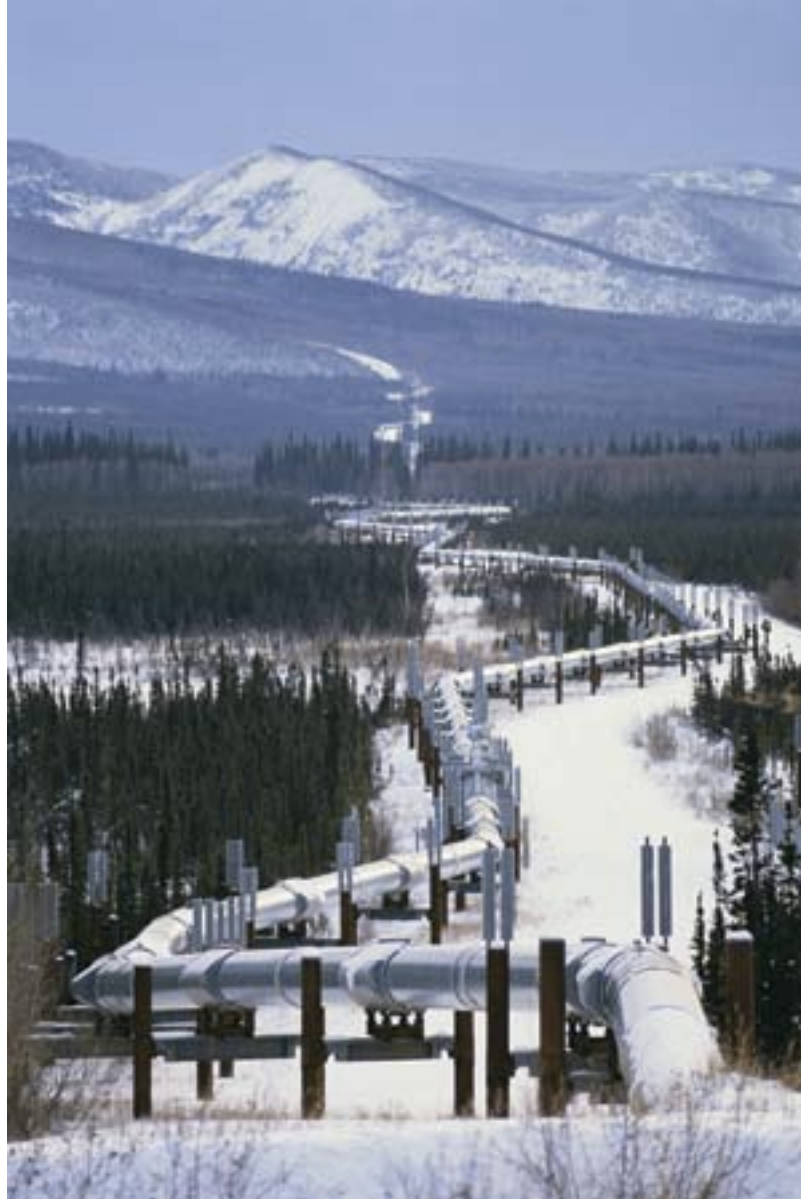
Trans-Alaska Pipeline: 800 miles (1290 km), 48 in. (1.2 m) diameter Pipe wall thickness ~0.5 in. Takes oil 11.9 days to travel the length at an average speed of 3.7 mph (6.0 kph)
