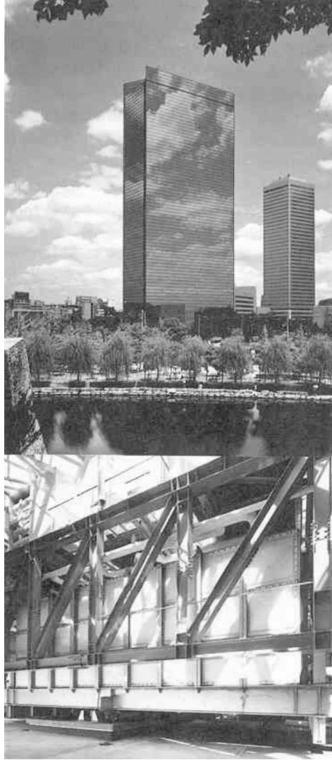
FIGURE 4.11: Ice storage tank—Crystal Tower. (Courtesy of Takemaka Corporation.)
